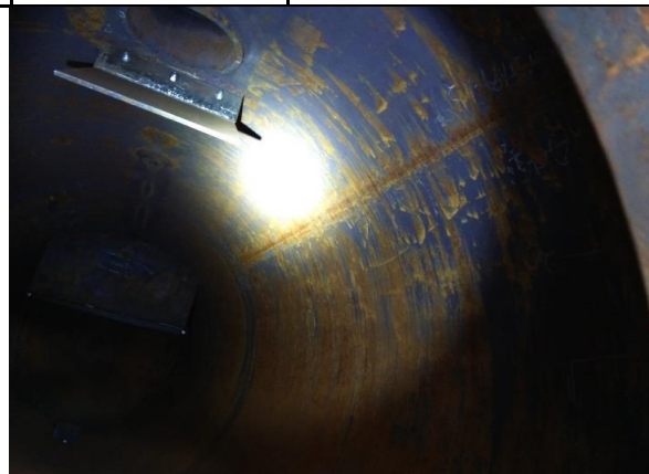
Photo 12 Description: Internal inspection, slight surface rust
