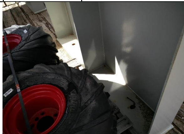
Photo 18 Description: Anchor bolt holes
