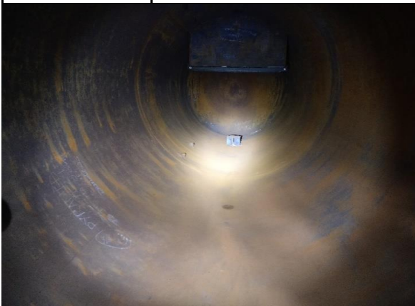
Photo 11 Description: Internal inspection, slight surface rust
