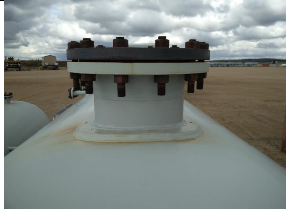
Photo 14 Description: Split repad on nozzle weep hole still grease
