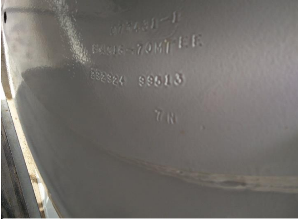
Photo 7 Description: Manway split repad stamping
