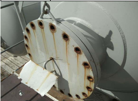
Photo 5 Description: Manway cover
